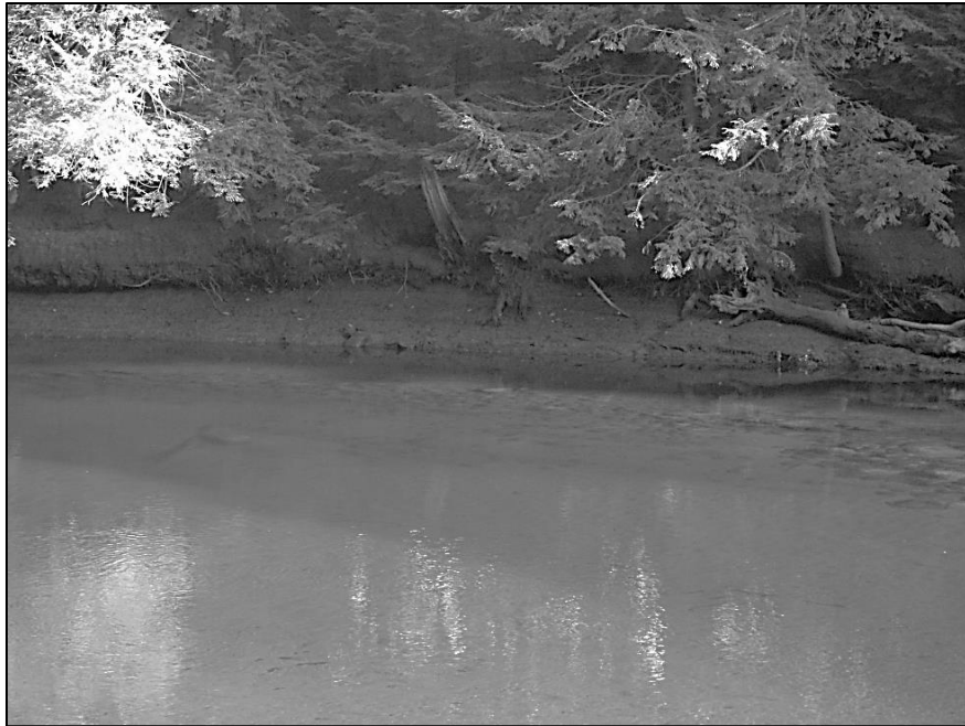
Figure 5. Eastern edge of dam, with dense conifers over sloping bank in background.
